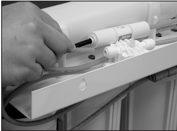
Figure 9 - Disconnect pre-carbon outlet tube from shutoff valve
